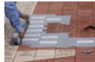
Taped down with duct-tape to avoid damaging neighboring bricks.
