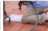
Sandblasting the letters through the template into the bricks.
