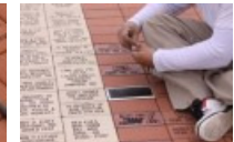
Carefully removing the remnants of the template.
