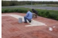
Laid out on the proper location.
