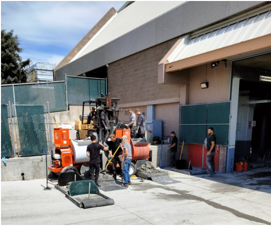
Mixing the Clay for the courts
